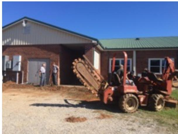
Heavy equipment was needed to run underground electrical lines for the air conditioning units.
